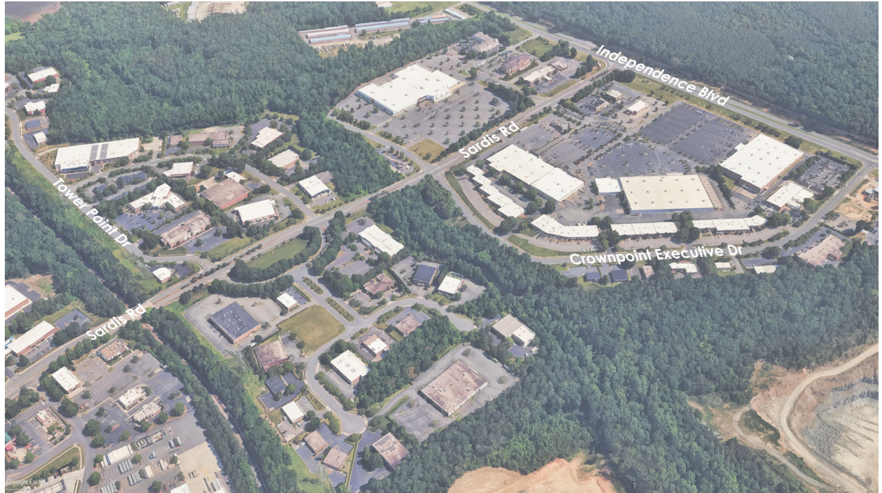
FIGURE 11: AERIAL OF EXISTING CONDITIONS
